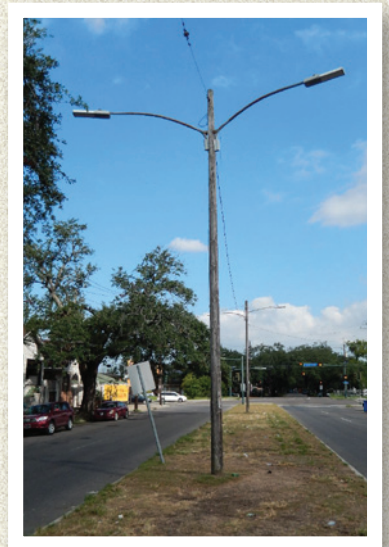
Modern LED Lighting
